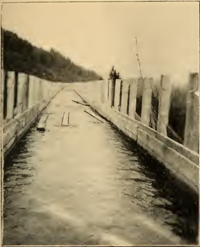
SHOWING FLUME CONSTRUCTION.
